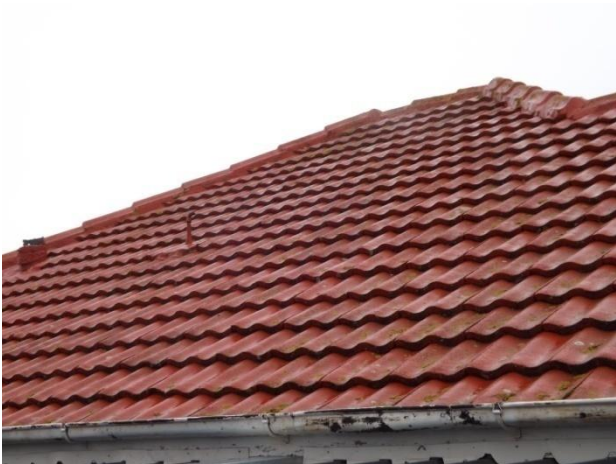
Tile roofing secure.
