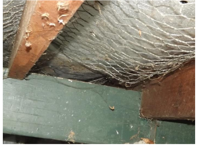
Sub-floor to extension secure.
