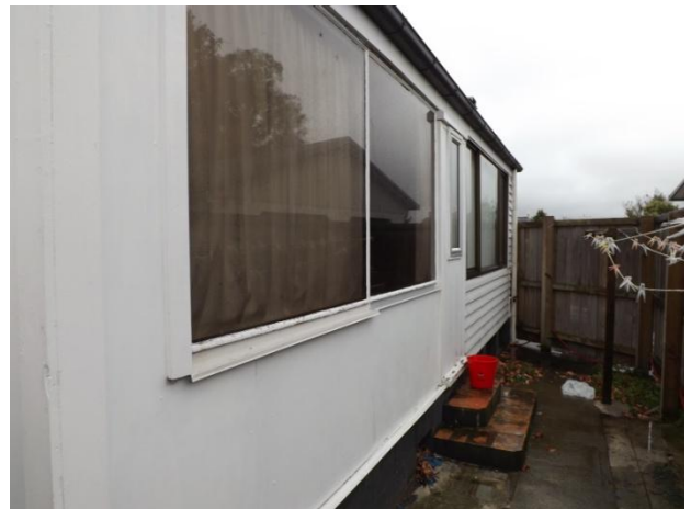
Extension to east.
