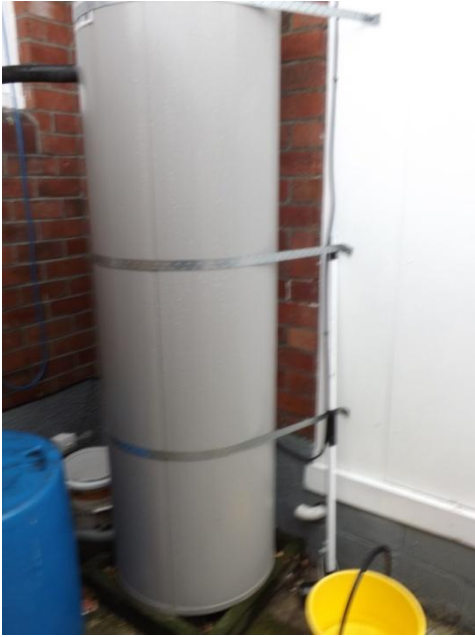
Secure hot water cylinder.
