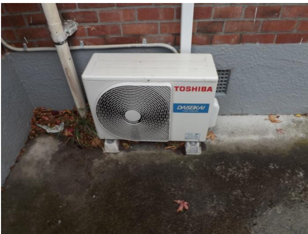
Insecure heat-pump.
