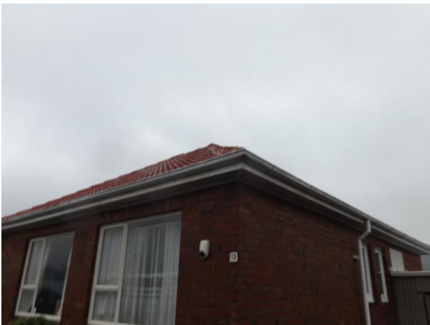
South/east hip blade is sagging.
