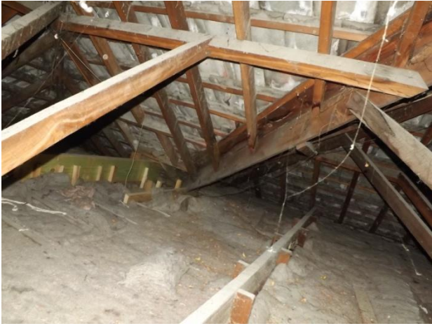
Insulation well-placed; new ceiling beam well-built over lounge area.
