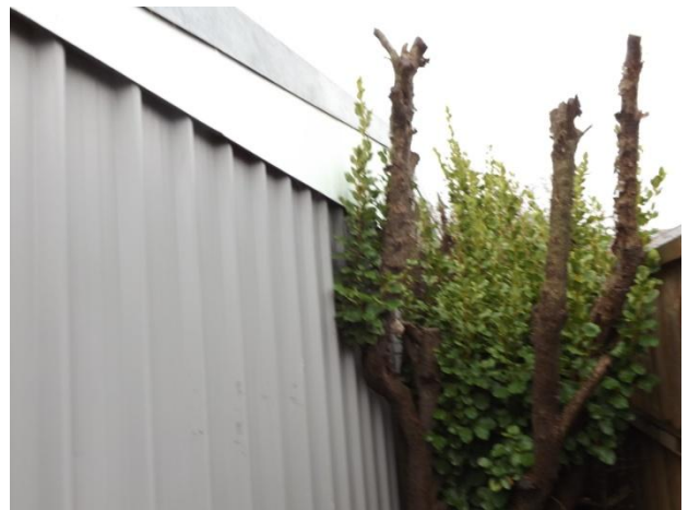
Rear of garage in good order.
