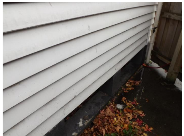
Borer to cladding.
