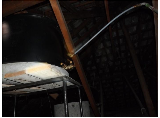
Water-tank in roof-space not secured.
