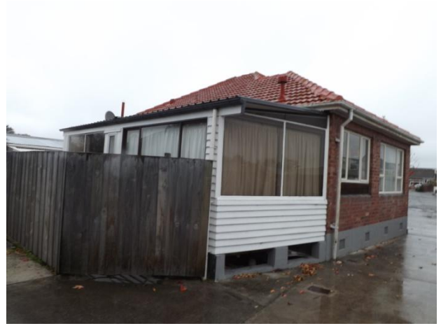
New extension to east elevation.
