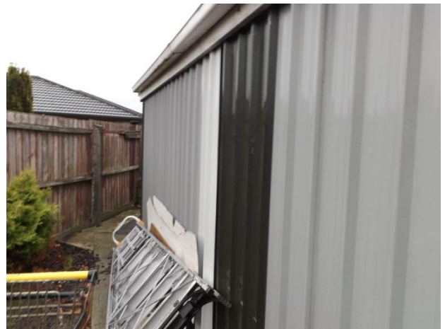
Secure side of garage cladding.
