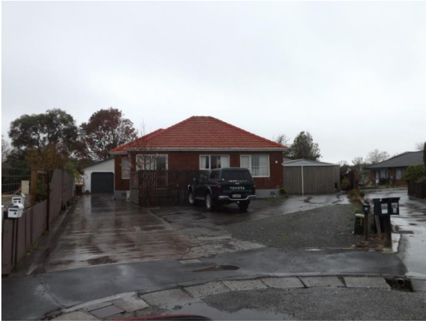
West elevation to road.
