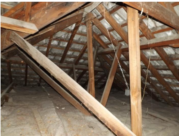
Secure roof framing.
