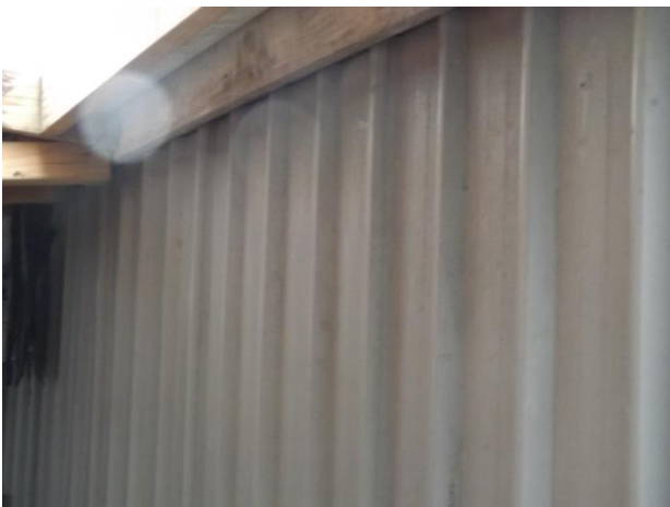
Secure shelter to south elevation.
